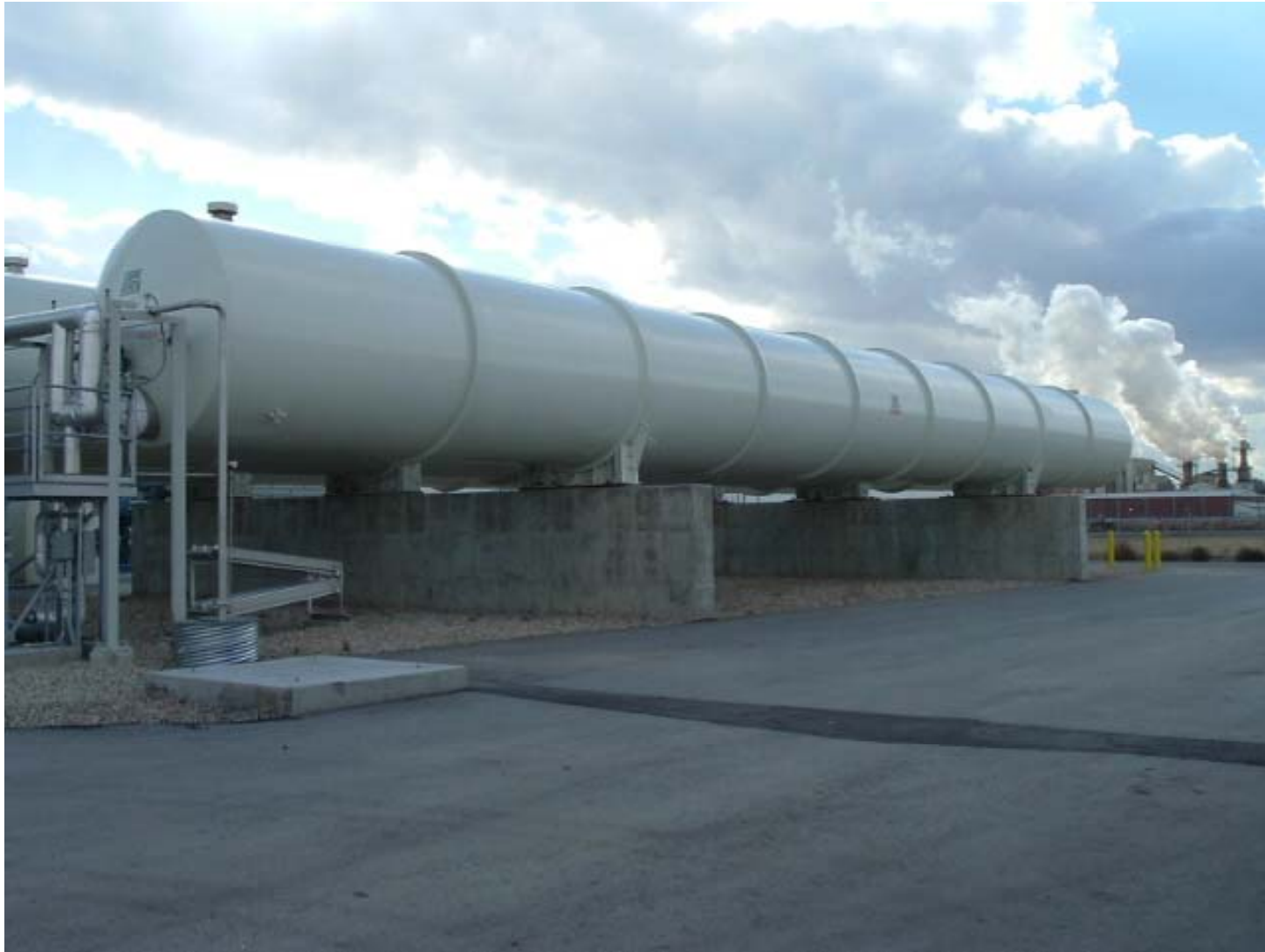
Figure 35. 50,000 gallon liquid oxygen storage tank.
