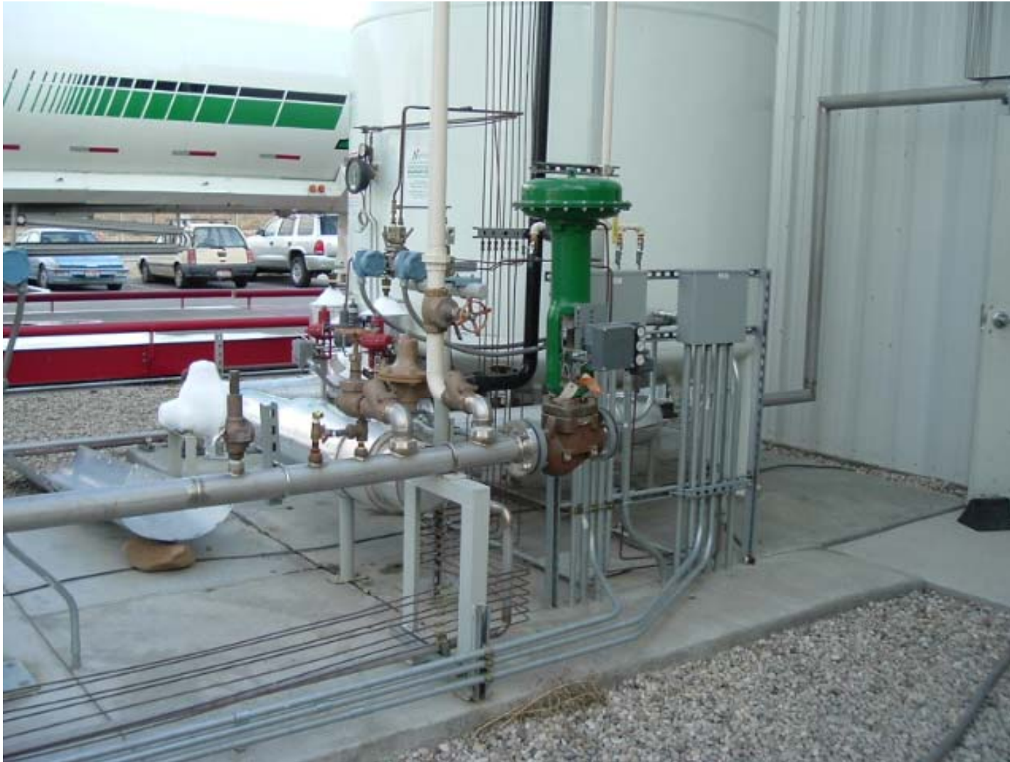
Figure 37. Oxygen gas regulator assembly.
