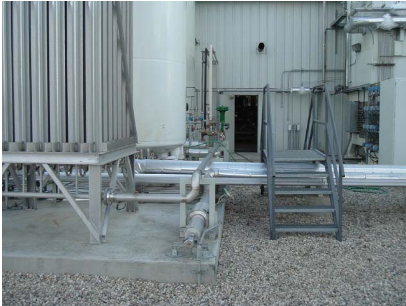
Figure 36. Vaporizer/discharge piping.
